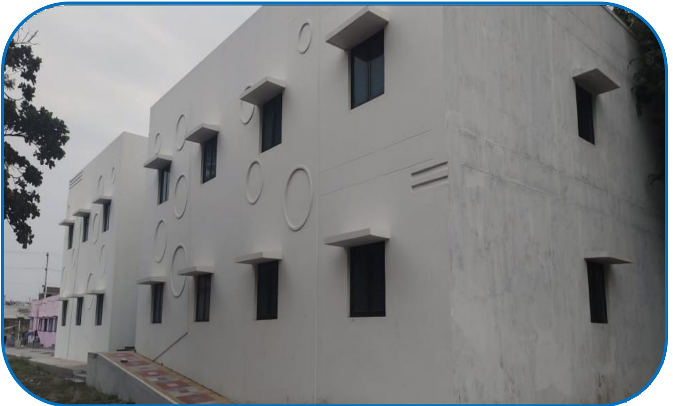
LIBRARY BUILDING (G+1)
